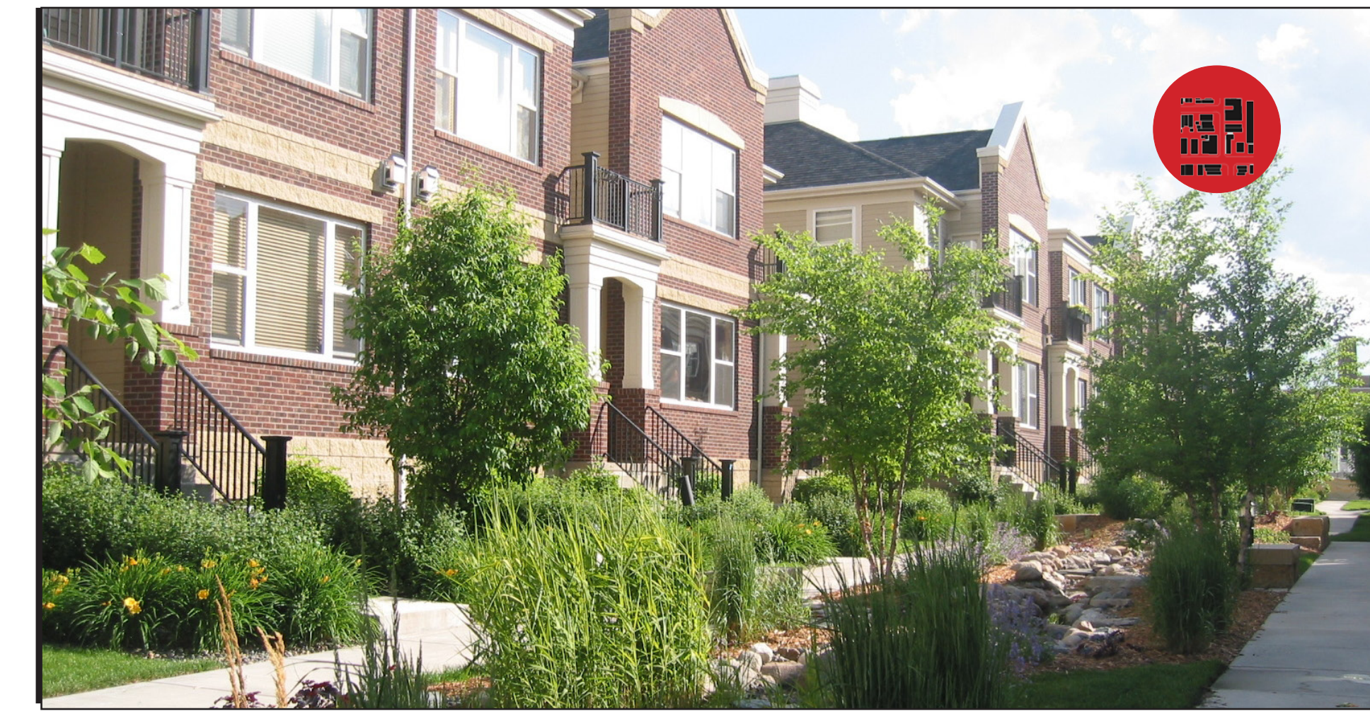
Implement strategies detailed in the current Wellhead Protection program to create awareness of groundwater protection
