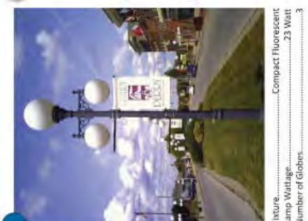
Fixture.....Compact Fluorescent Lamp Wattage.....23 Watt Number of Globes.....5
