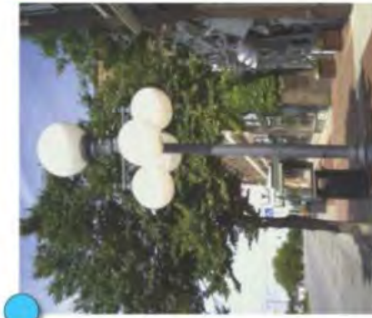
Fixture.....Compact Fluorescent Lamp Wattage.....23 watt Number of Globes.....5
