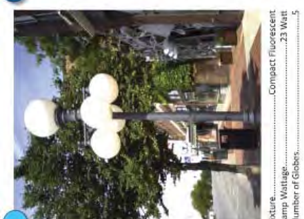
Fixture.....Compact Fluorescent Lamp Wattage.....23 Watt Number of Globes.....3
