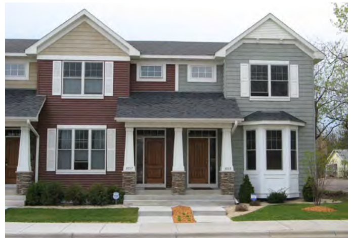
Single-family attached housing in the 1st Avenue Corridor Activity Center can provide a nice transition to adjacent single-family neighborhoods and diversify the housing types available in Perry.
