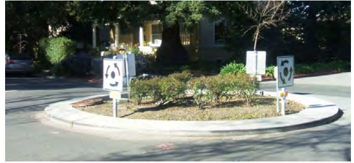
A traffic circle slows drivers, a strategy more appropriate for local, collector, and in some cases minor arterial streets.
