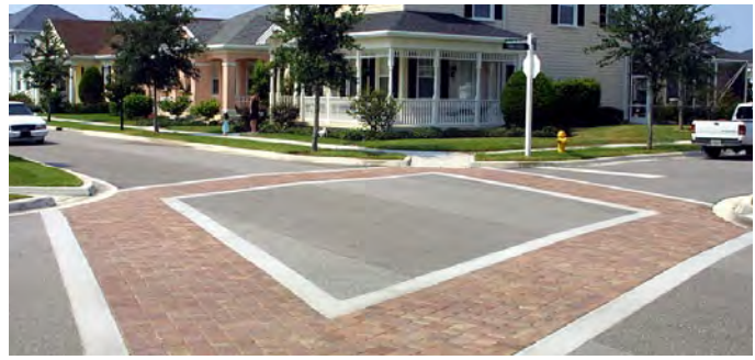
An intersection with crosswalks that use alternative pavement calls attention to the pedestrian realm.
