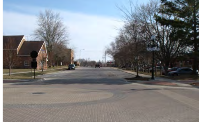
Downtown streetscape enhancements include bumpouts, pedestrian scale lighting, colored pavement, decorative fencing, and street trees.
