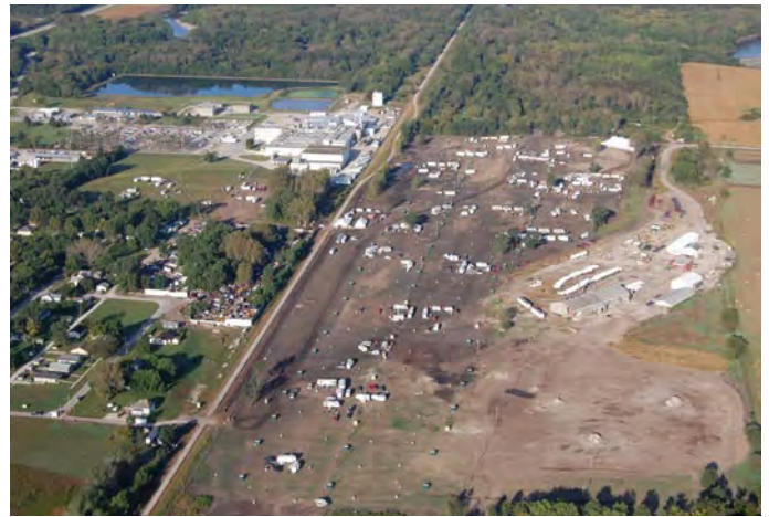
Existing brownfield site to be cleaned up in next few years
