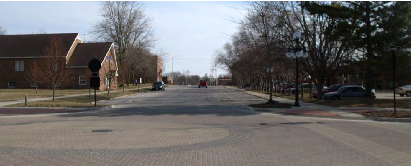
Distinctive paving patterns such as the 3rd and Lucind Street intersection create an attractive intersection and improve the pedestrian experience.
