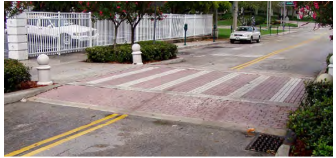
A speed table provides a more distinct pedestrian crossing, slows traffic, and reduces the pedestrian crossing distance.
