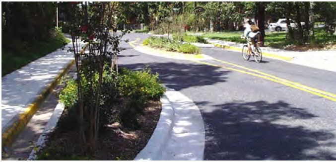
A street altered with landscaped bump outs varies the travel lane and slows traffic.
