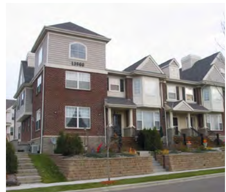
Multi-family residential developments should include features such as individual entrances, porches, and gables.
