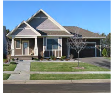
Subdivisions should have sidewalks and homes with design features that minimize the presence of the garage along the street.
